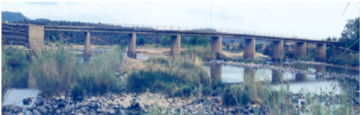
Figure 4 Photograph of bridge profile plotted in Fig. 3, facing downstream
