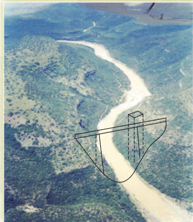
Aerial view of dam site at Jana
