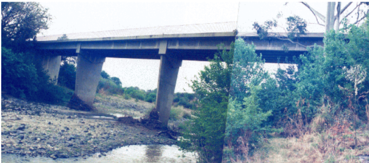
Figure 6 Photograph of bridge across the Bushmans River, facing downstream
